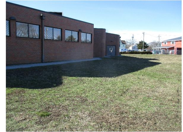
Three bioretention system locations have been identified around the north side of the building which can capture and infiltrate stormwater runoff from the rooftop of the building. A preliminary soil assessment suggests that more soil testing would be required before determining the soil's suitability for green infrastructure.
